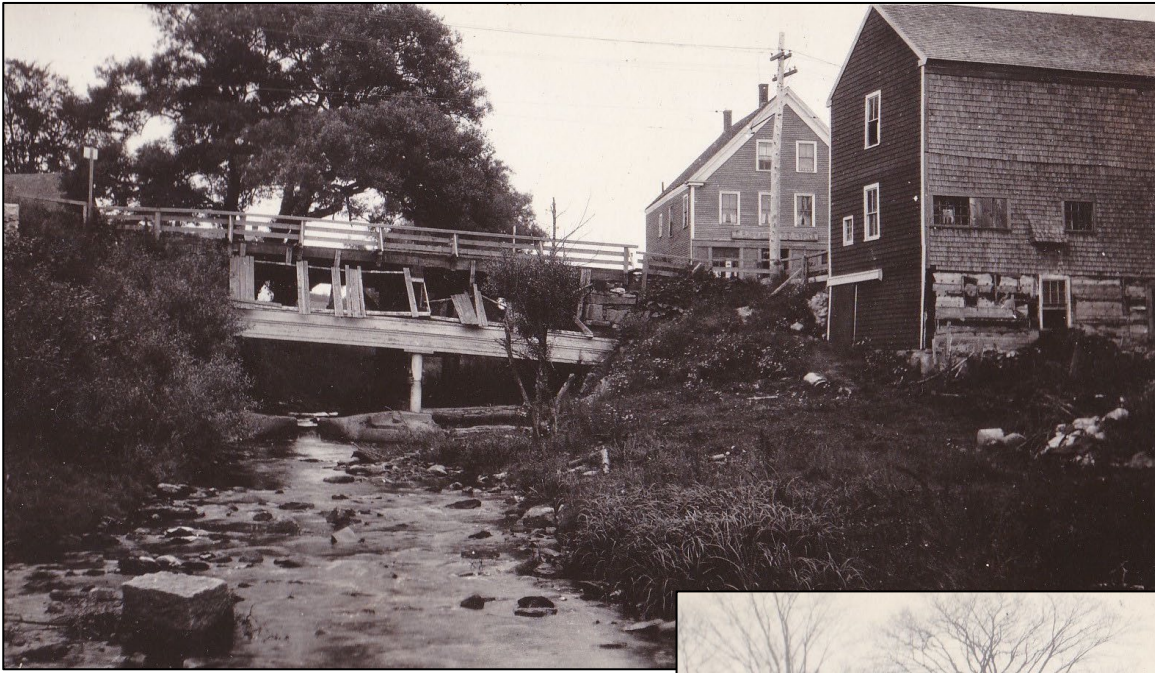
Looking north from below the old bridge before culvert and fill were added in 1923/24
